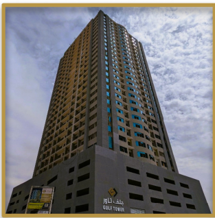
Gulf Tower BMS Upgrade
